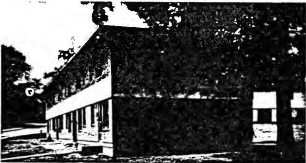
Children playing on the unkept grounds of America Park (top). Those units with the least disrepair (middle) were repaired and maintained for use until the completion of the new development (bottom).
